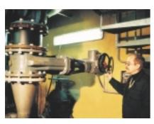
Installing MSF Soft Starters to control pumps resulted in several benefits for the Boden Municipal waterworks in Sweden. Gradual stopping of a high-pressure pump prevented water hammer, thereby prolonging its operational lifetime significantly. Since the pump starting current was reduced by more than 50 %, the main fuses could be downsized. And motor-operated valves could be replaced by ordinary reverse valves. These benefits resulted in savings of Euro 6 000 for pump renovation.
