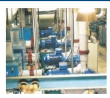
Imperial Tobacco of Nottingham, England, installed larger condenser pumps to drive the chillers of their upgraded air-conditioning plant. As any three pumps can be started simultaneously, a control system was needed to prevent uncontrolled current inrushes, initial high torque, and water hammer when stopping pumps. This is why MSF Soft Starters were chosen.
